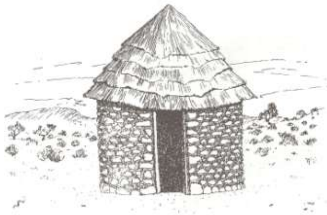
Figure 1: A rondavel built of earth and stone.
